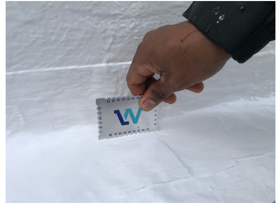
Figure 16: verify first resin application is 45 mils wet thickness (min)
