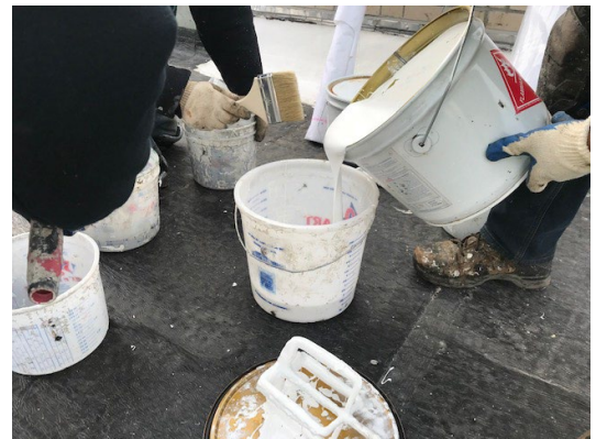
Figure 12: use and catalyze what is needed for the installation.
