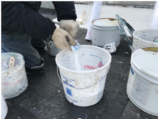
Figure 13: add PMMA catalyst as required to PMMA resin.
