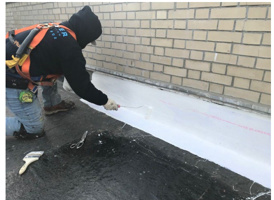
Figure 20: saturate fleece reinforcement with 2 nd PMMA coat.
