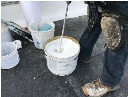
Figure 11: mix-agitate PMMA resin.
