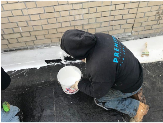
Figure 15: apply to prepped and primed substrate with roller.
