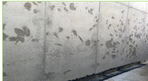
Figure 8: acceptable grout filling and fin removal
