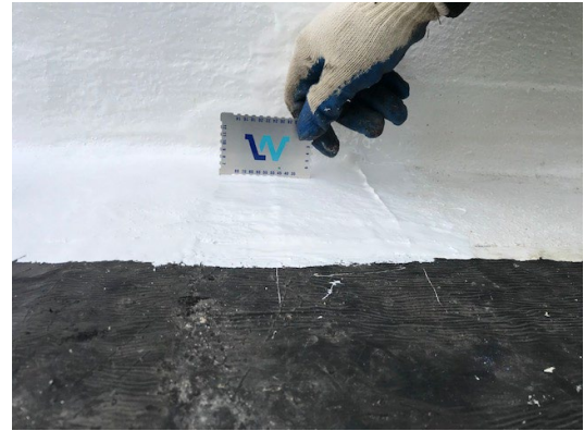
Figure 22: verify 2 nd PMMA resin coat is minimum wet 45mils thick.
