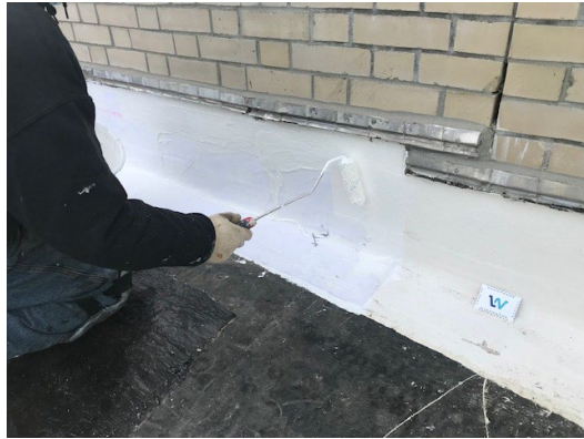
Figure 21: overlap 2-inches on existing PMMA as required.
