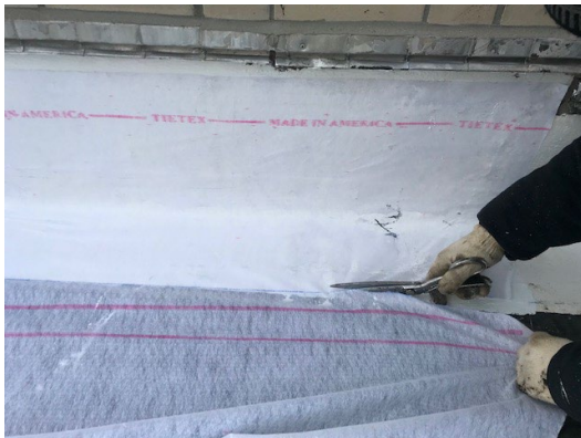
Figure 19: cut leading edge of fleece 1/4-inch from edge of resin.
