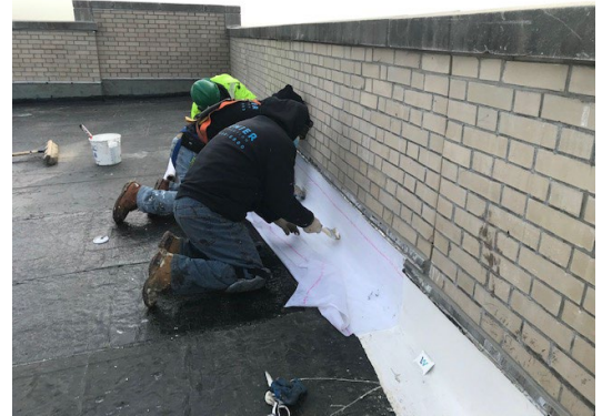
Figure 18: set fleece reinforcement into fresh PMMA resin.
