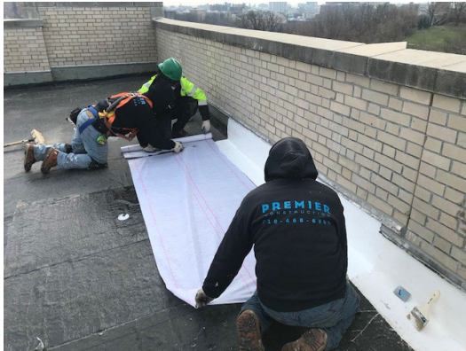
Figure 17: install fleece reinforcement.
