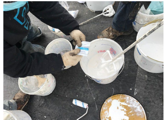
Figure 14: thoroughly mix and evenly disperse catalyst into resin.
